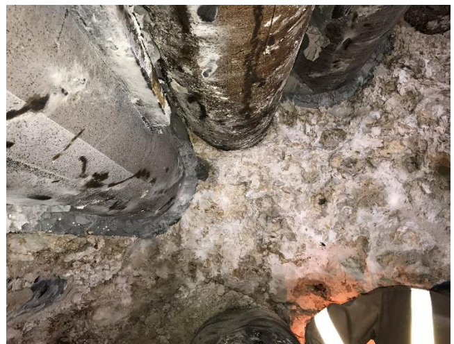
only 20 mm tolerance in the pipe arch, anulus was grouted
