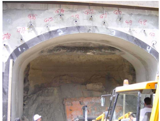
after grouting, excavation with a JCB
