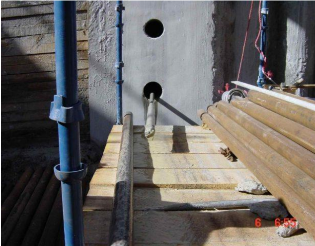
all 508 bores with a measurement tolerance of less than 3 cm at a depth of up to 8 m
