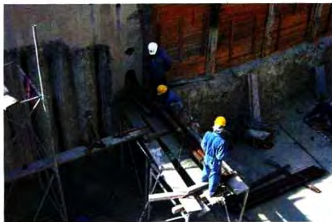
Sectional construction of the tunnel after the injection bores.
